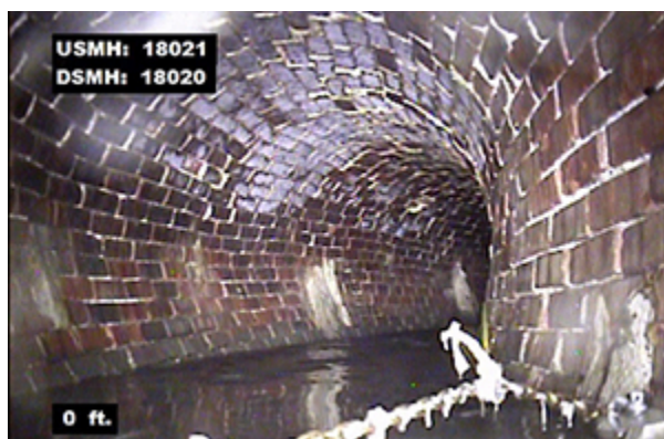
Brick storm sewer pipe
